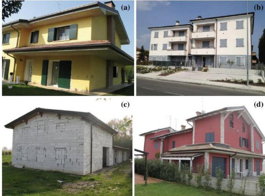
**Fig. 15** Examples of undamaged buildings: **a** two-storey unreinforced clay masonry building in Casoli di Sopra, municipality of Finale Emilia; **b** three-storey reinforced clay masonry buildings in S. Felice sul Panaro; **c** single-storey unreinforced masonry building with AAC units in Carpi; **d** four-storey reinforced masonry building with LAC units in Vigarano Mainarda
