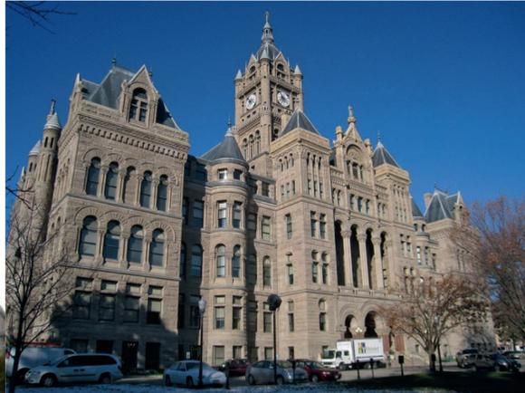
Salt Lake City and County Building, Utah, USA. The first building to be retrofitted using seismic isolation
